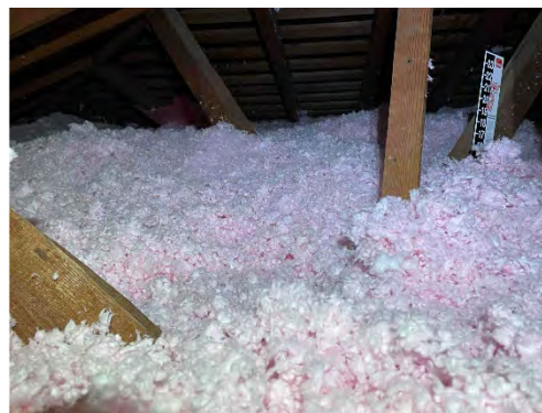
Attic cleaned and new insulation installed in parsonage.
