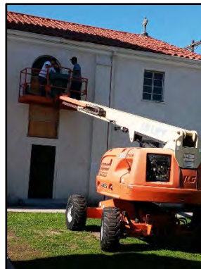
Step 2: Re-Install Stain Glass
